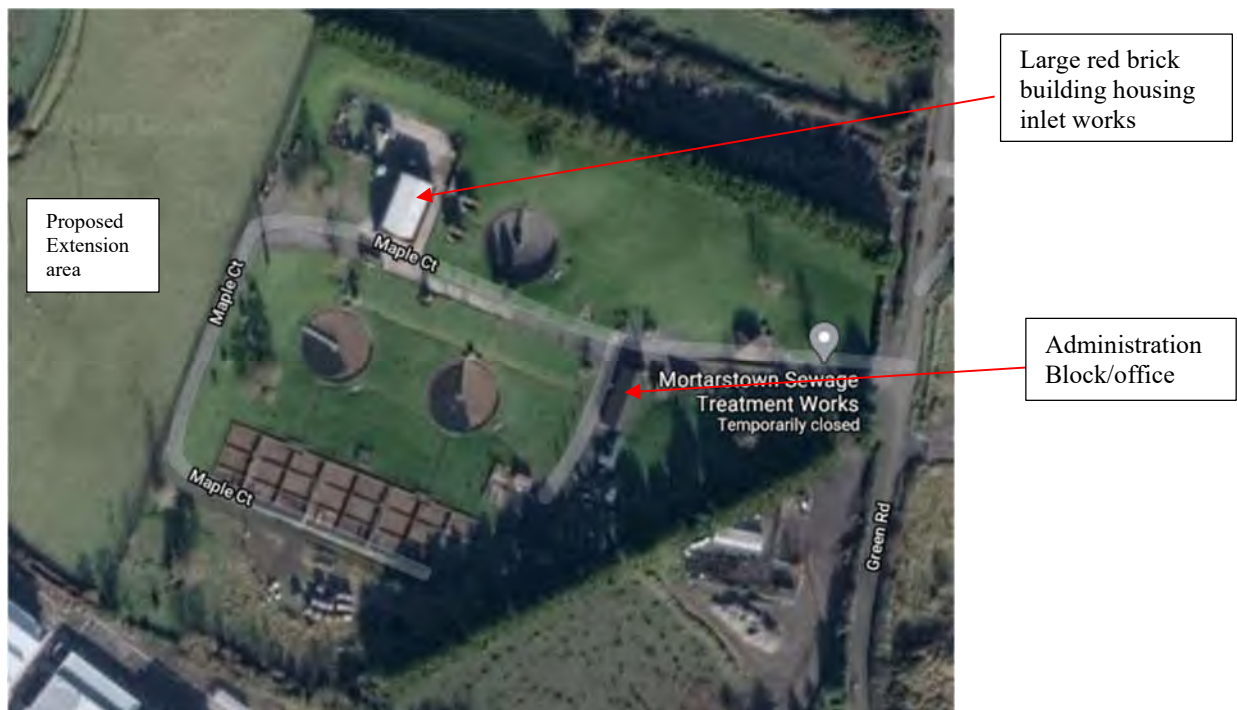
Figure 1 – aerial view of layout of Mortarstown Waste Water Treatment Plant and proposed extension area to the west of the existing site.
