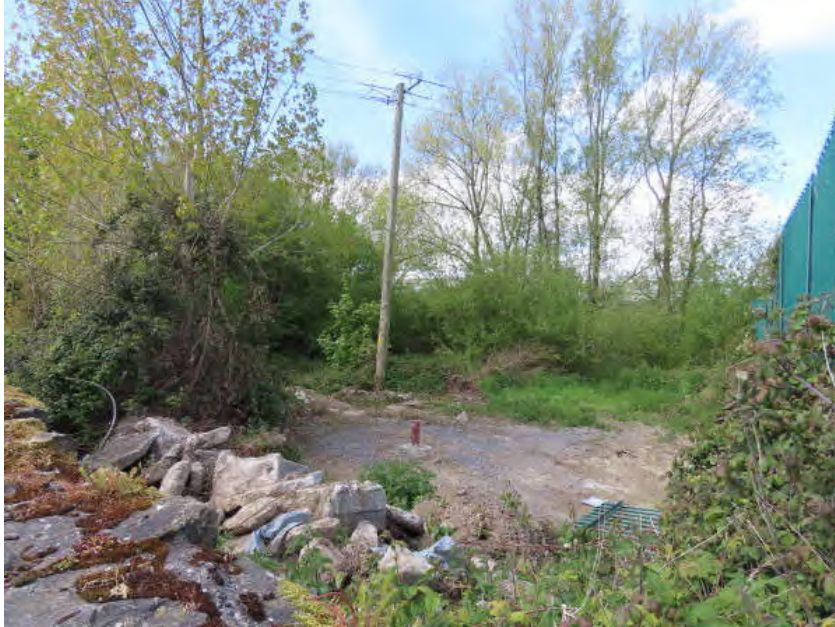
Photo 11 – area to south of Pumping Station for proposed extension
